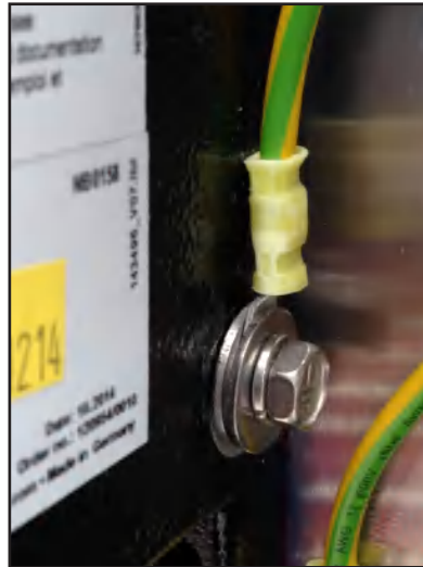
Figure 3 Earth Bolt And Nut Washer Assembly
