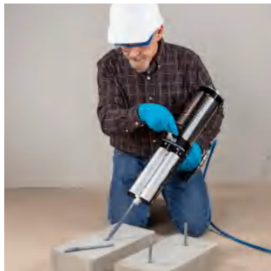
Powerful 2K pneumatic dispense guns are ideal for crack injection applications.
